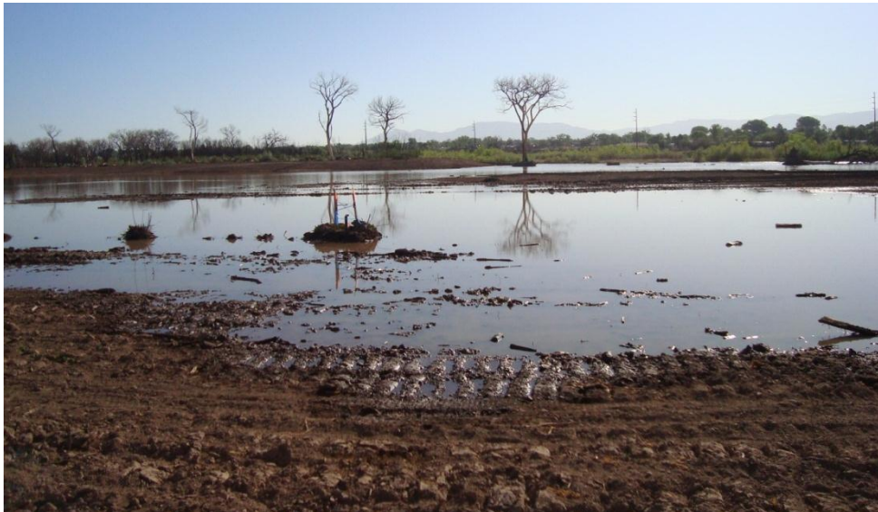
Picture 4. May 7, 2009: As Rio Grande flows reach 2,500 cfs they start to flow into the new backwater area. North well was left on an island of unlowered land to protect the well.
