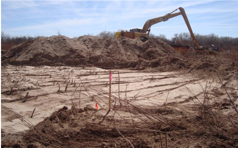
Picture 3. March 2009: Marsh buggies were used to lower the backwater area by 2 to 4 feet.
